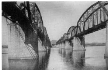
Railroad Bridge over Han River
